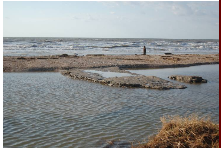
Figure 4: Remaining beach along Highway 87 near High Island, TX. Clay outcroppings exposed.
