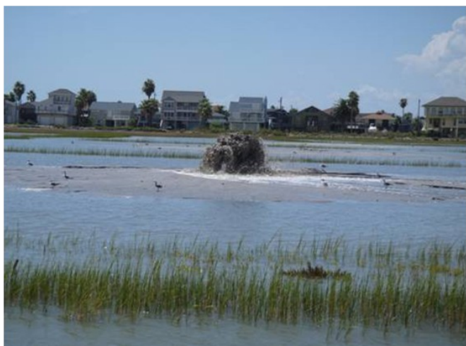
Fig. 1. Dredged material being discharged for marsh mound creation.
